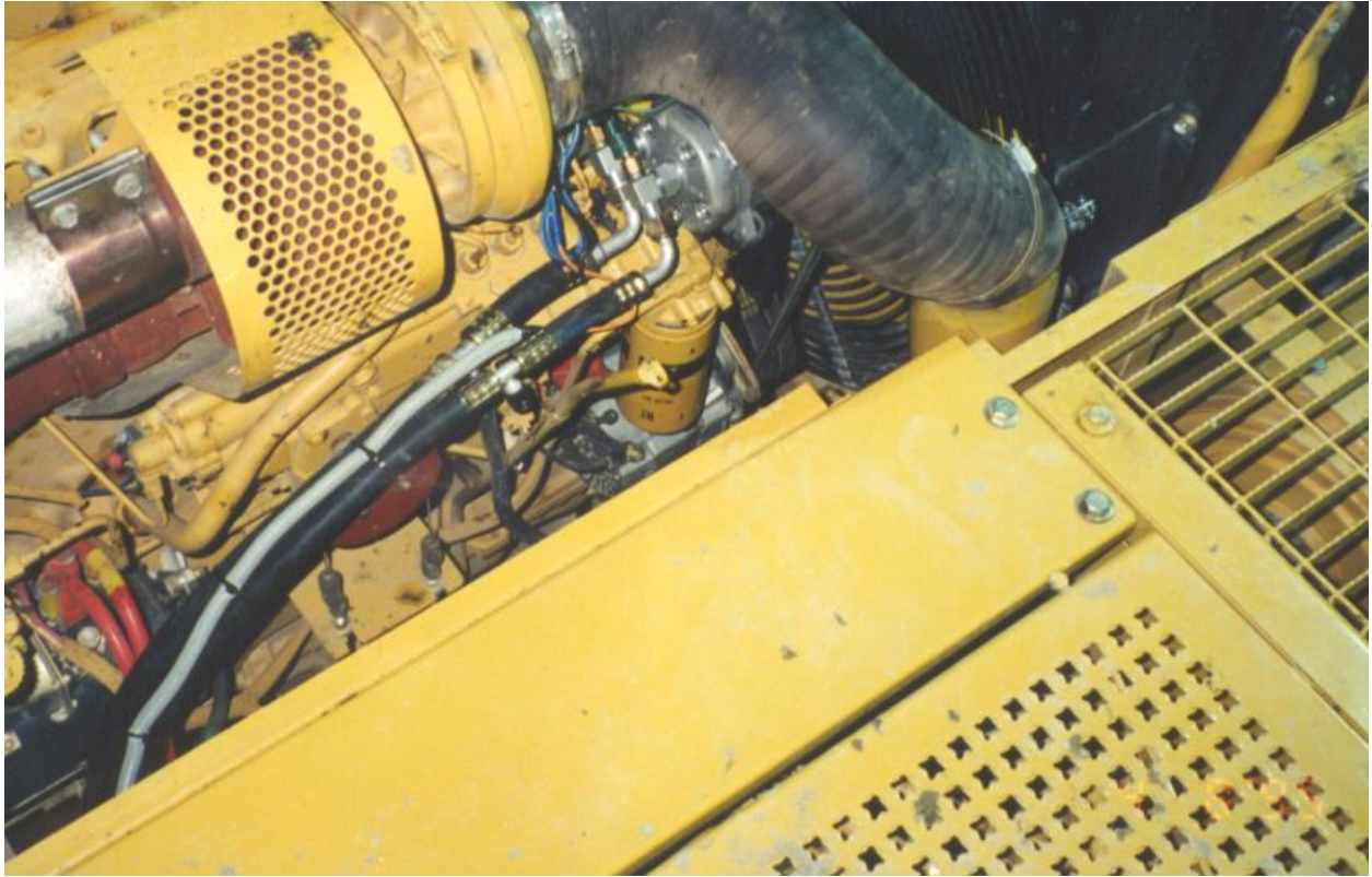
Rear view of compressor in place with hose routing.
