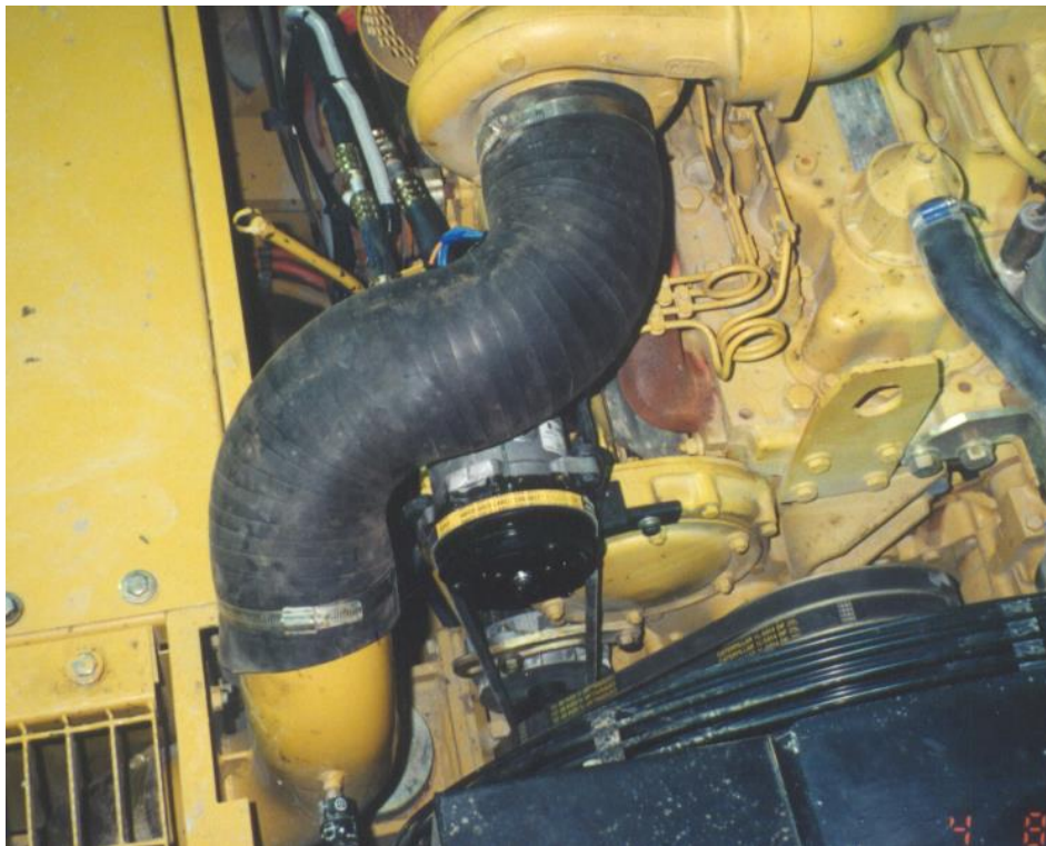
Front view of compressor in place.
